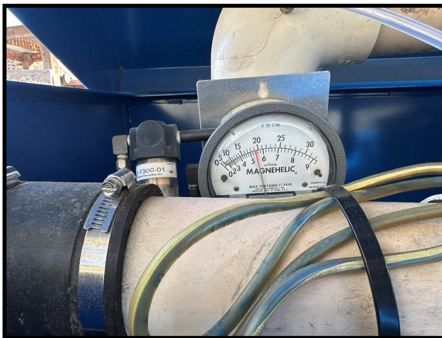
Photograph 19 – Flow Rate through Blower Motor after Well Adjustment
