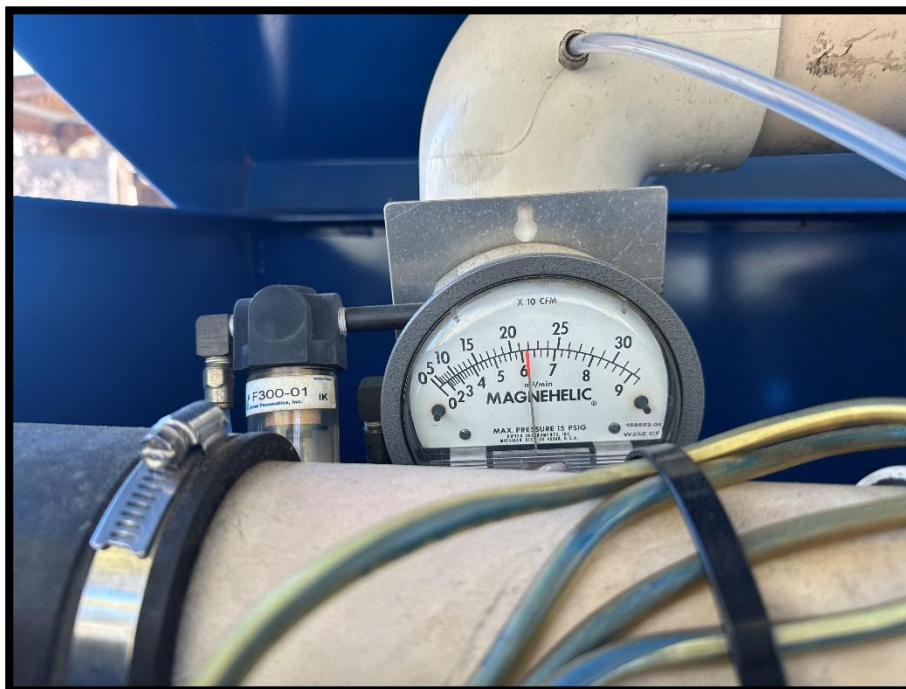
Photograph 18 – Flow Rate through Blower Motor before Well Adjustment
