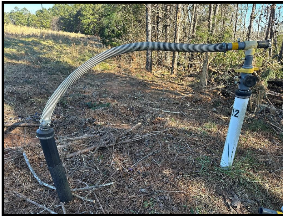
Photograph 23 – Repaired Extraction Well 12
