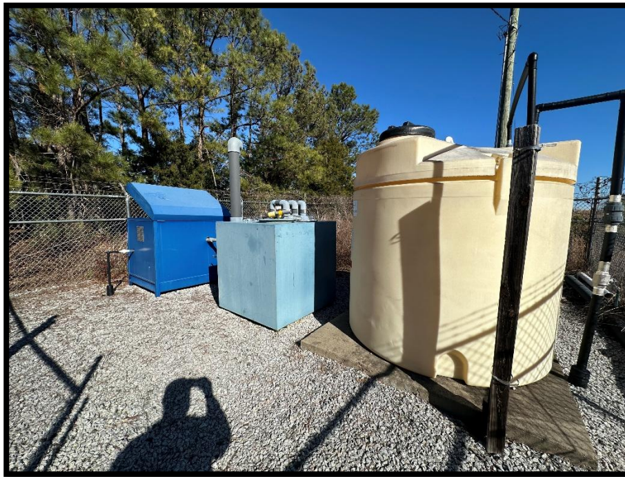
Photograph 21 – Soil Vapor Extraction System
