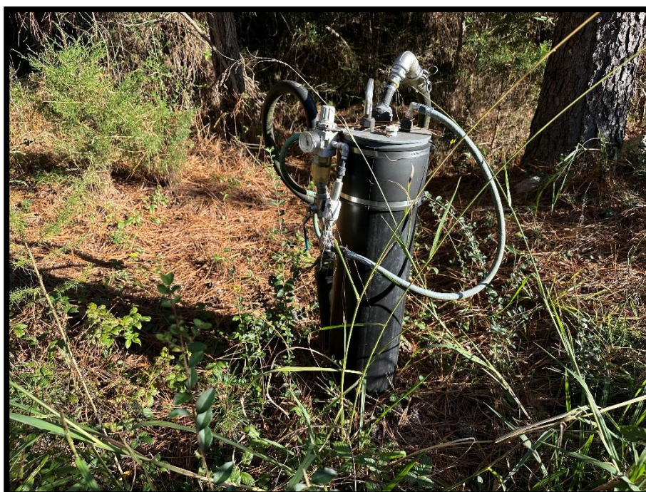
Photograph 12 – Condensate Pump C
