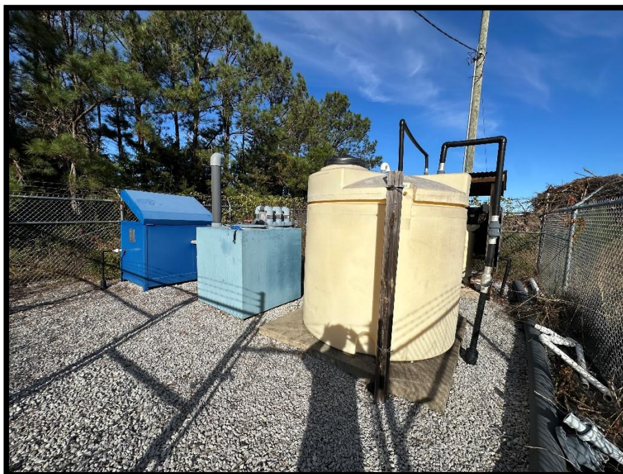
Photograph 20 – Soil Vapor Extraction System
