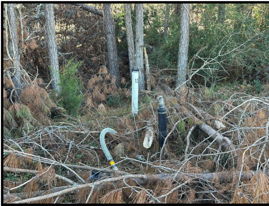
Photograph 21 – Damaged Extraction Well 12
