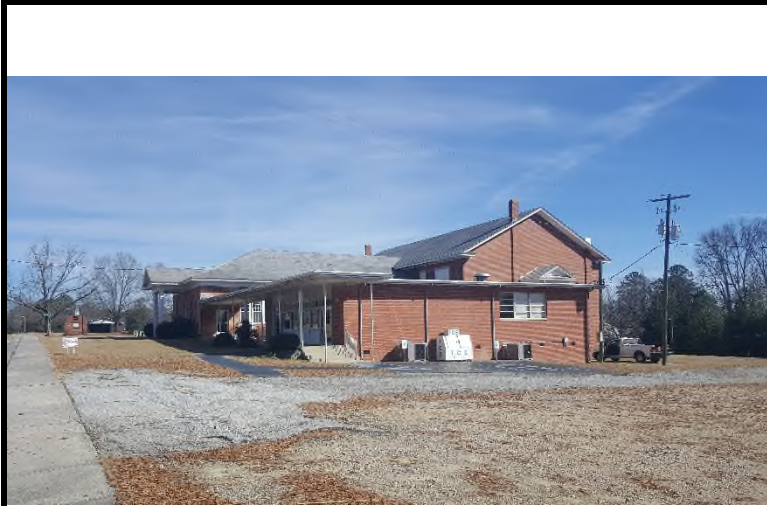
1 General view of the subject building. The cafeteria building in the foreground with the flat roof was not included in the assessment.
