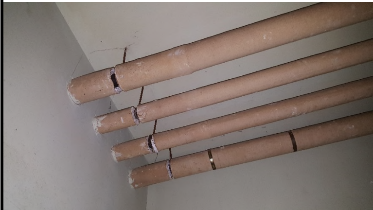
7 The pipe insulation by the ceiling in the basement contains asbestos (20% amosite, 15% chrysotile).
