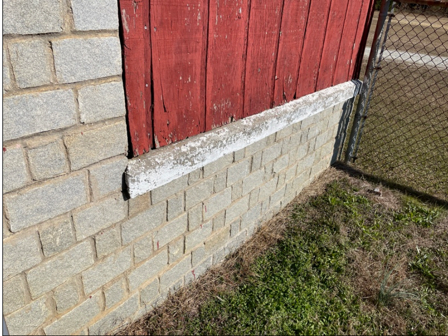
11 - White LCP on Concrete Trim of North Barn
