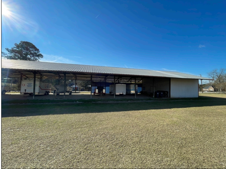
1 - View of Carport/Training Center
