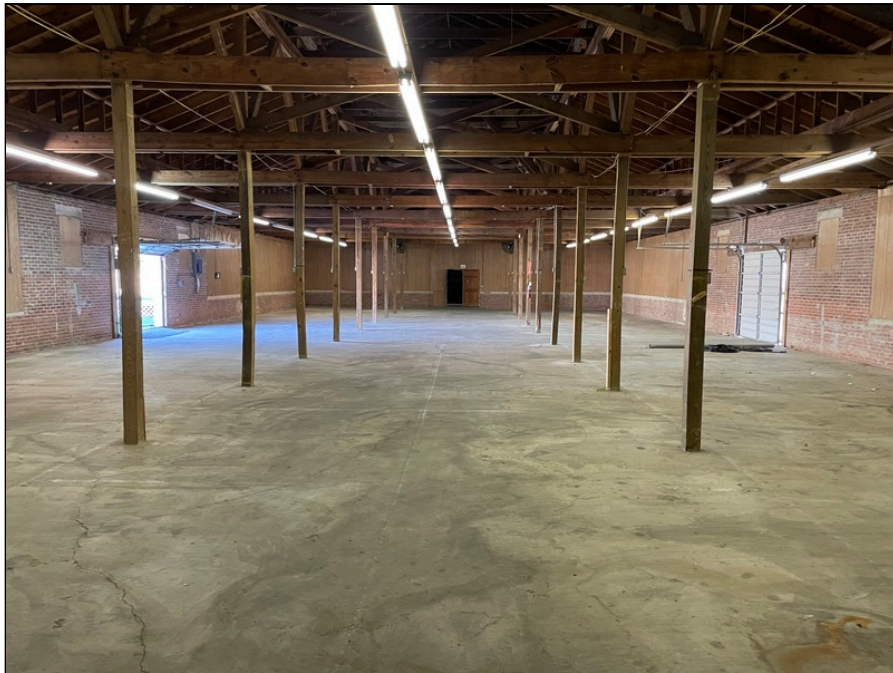
8 - South Barn Interior
