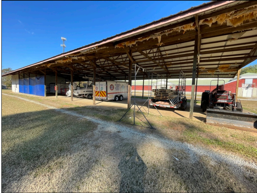
3 - View of Carport Area
