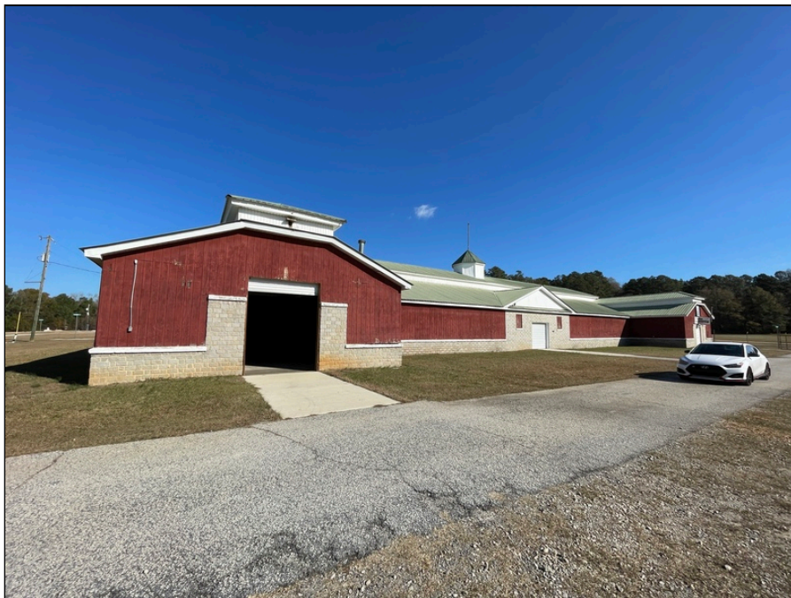
4 - View of South Barn
