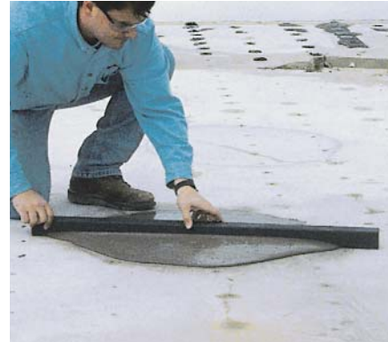
Screed Zono-Patch to a smooth finish.
