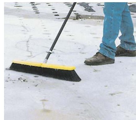
Remove all debris from the area.
