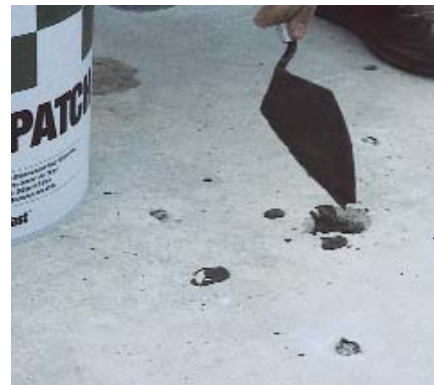
Fill and repair divots with a trowel.
