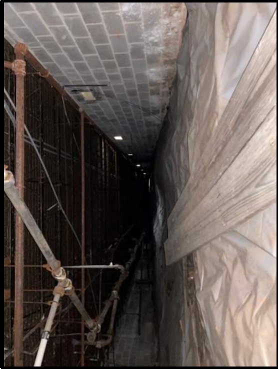
12 General view of crawlspace.
