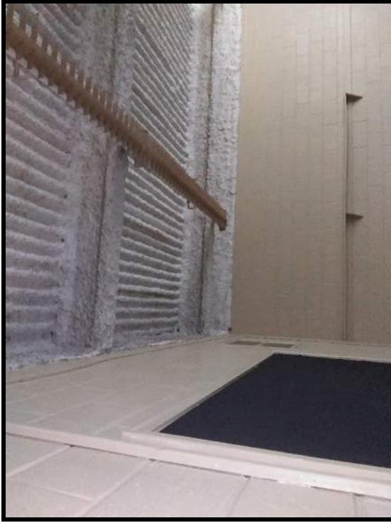
2 Spray-applied fire proofing tested negative for asbestos via PLM analysis.
