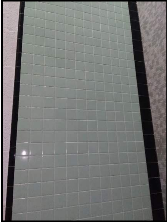
10 Green and black ceramic tile in men's restroom tested positive for lead based paint (5.40-19.90 mg/cm 2 ).
