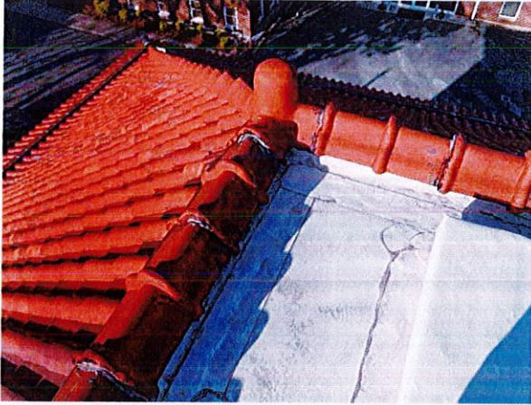
Repairs using sealants, mastics and coatings
