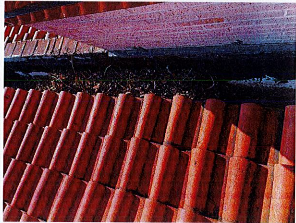
Debris in the built-in gutter system
