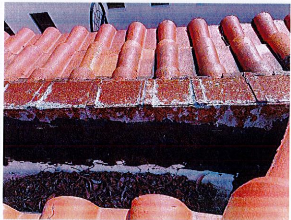
Substantial deterioration of the built-in gutter system
