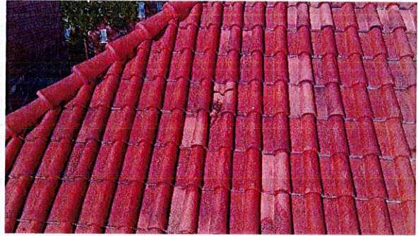
Broken and dislodged tiles
