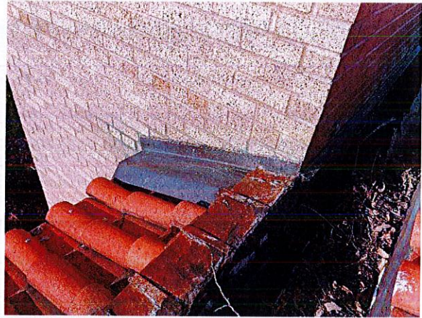
Dissimilar materials (steel and copper)
