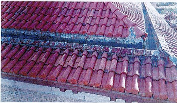
Repairs using sealants, mastics and coatings
