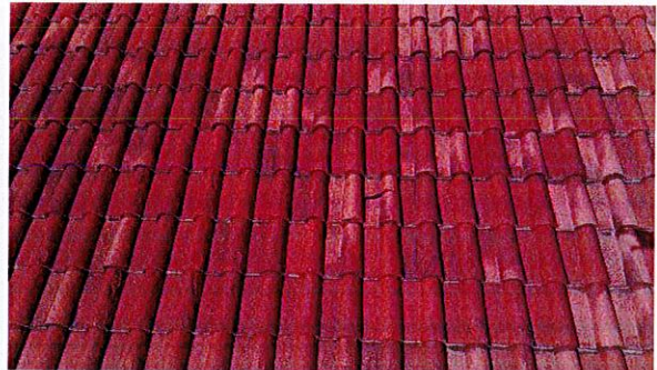
Broken and dislodged tiles
