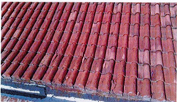
Substantial freeze/thaw damage to the clay tiles
