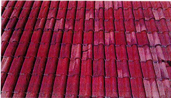
Broken and dislodged tiles
