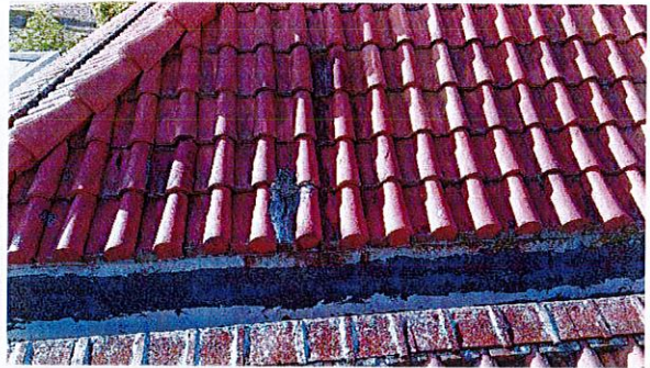
Repairs rmed using sealants, mastics and coatings
