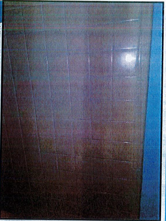
9 Yellow ceramic tile in men's restroom tested positive for lead-based paint (7.70 mg/cm 2 ).
