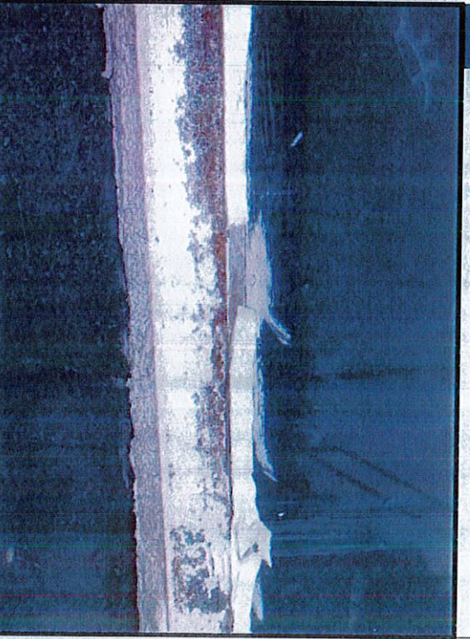
4 Window glazing tested positive for asbestos (2% chrysotile).
