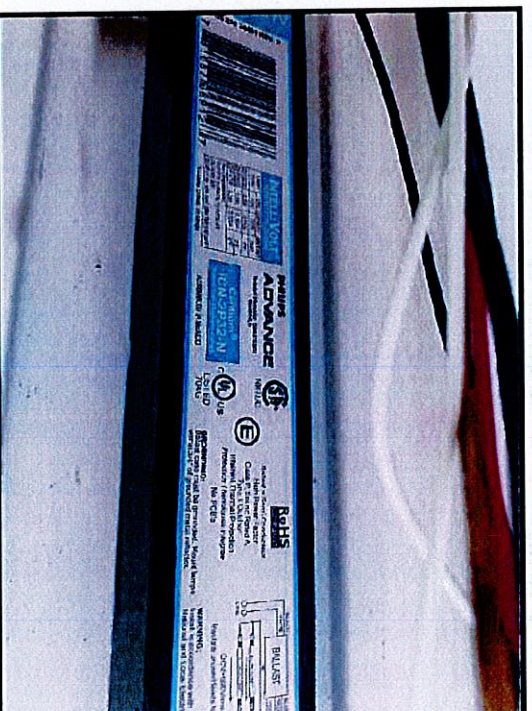
14 Ballast labeled no PCBs.
