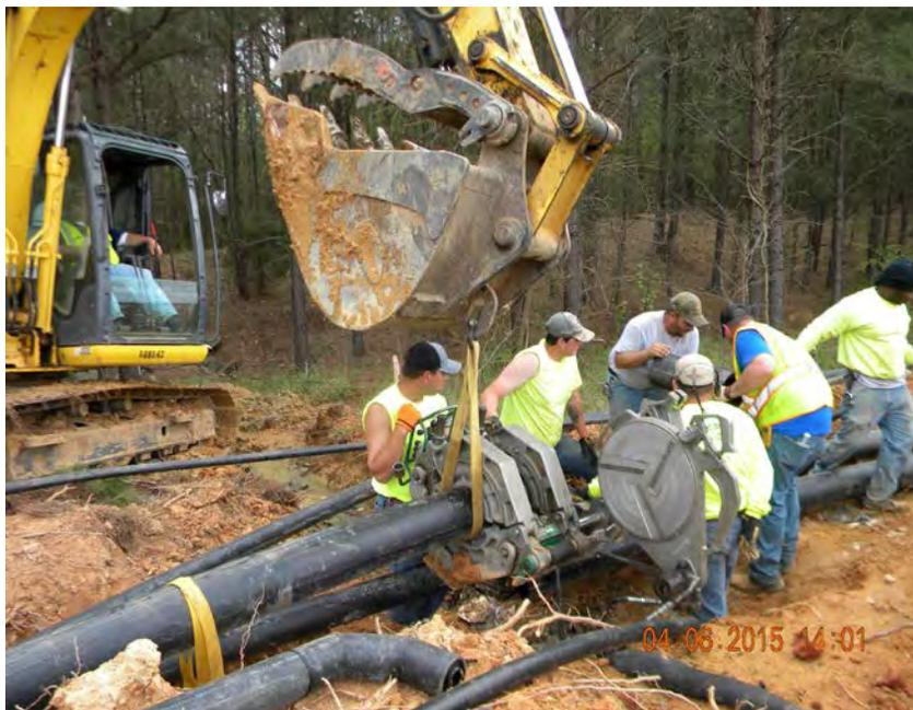
**Photo 4. HDPE pipe fusion welding machine**
