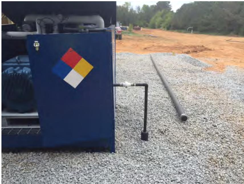
**Photo 18. Force main from knock out pot to storage tank.**
