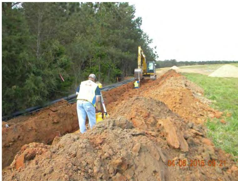
**Photo 8. Laser survey control for pipe**
