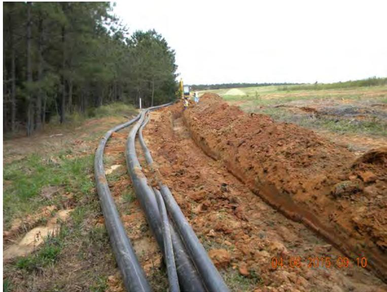
**Photo 5. Header trench and pipe**
