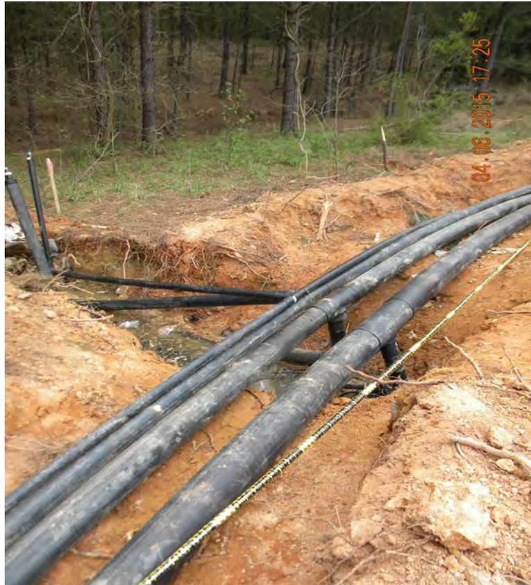
**Photo 7. Header pipe and lateral pipes to well**
