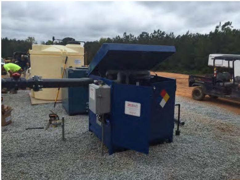
**Photo 15. Blower enclosure, vapor canister, and storage tank.**
