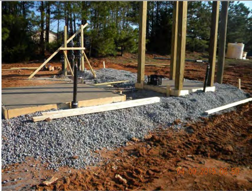
**Photo 13. Finished concrete pads for tank and air compressor.**
