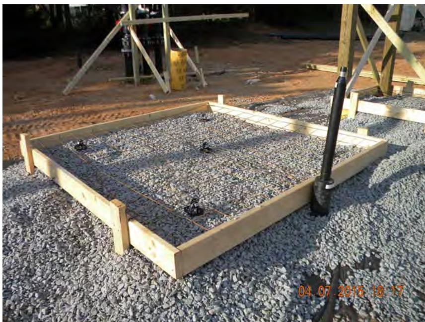
**Photo 12. Forms and wire mesh for storage tank pad**
