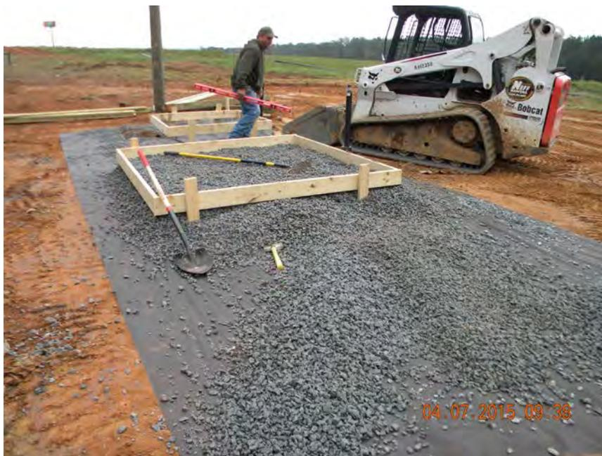
**Photo 11. Installation of forms and gravel pad**
