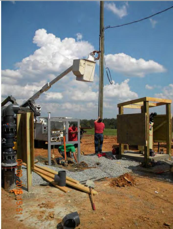
**Photo 14. Workers setting pole and electrical panel**
