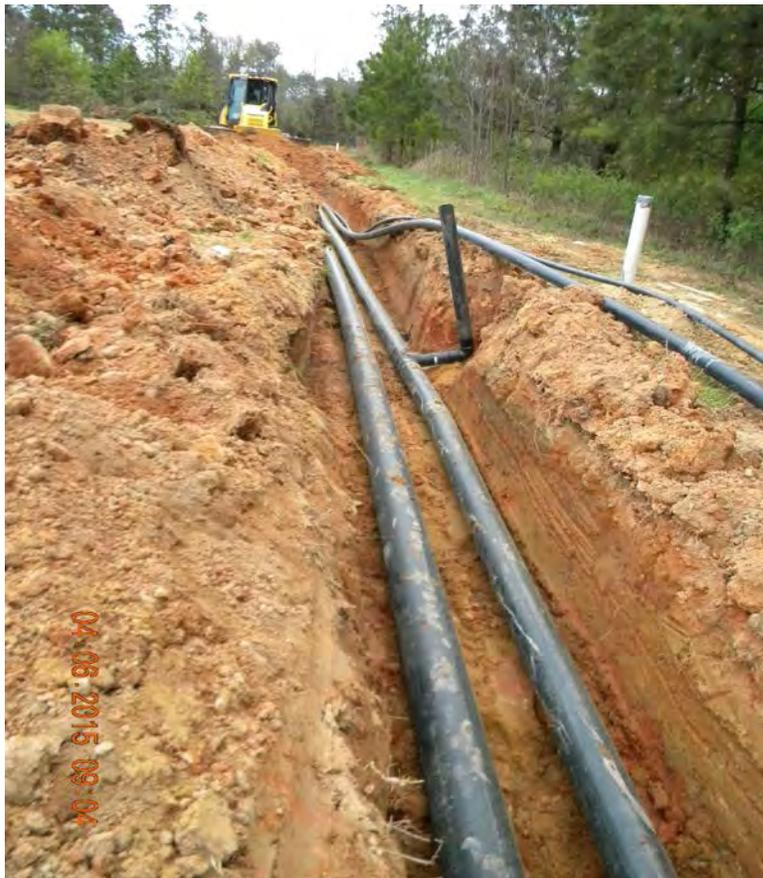
**Photo 6. Header pipe and lateral pipe to well**
