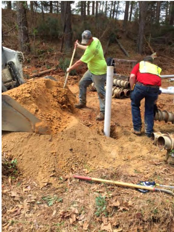
**Photo 3. Installing sand pack in well**
