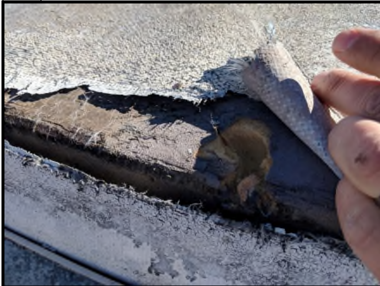
11 The cloth rolled roofing tested negative for asbestos.
