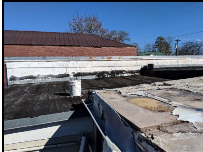
12 The asphalt rolled roofing tested negative for asbestos.
