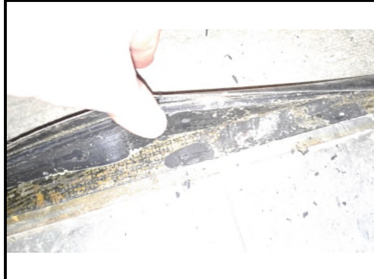
4 View of the black vinyl floor tile located beneath the 12" dark gray vinyl floor tile in the lobby and beneath carpeting in the clerk's office (10% chrysotile).
