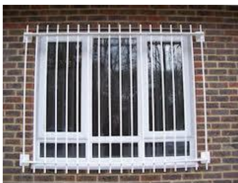
Bars and Grillwork
