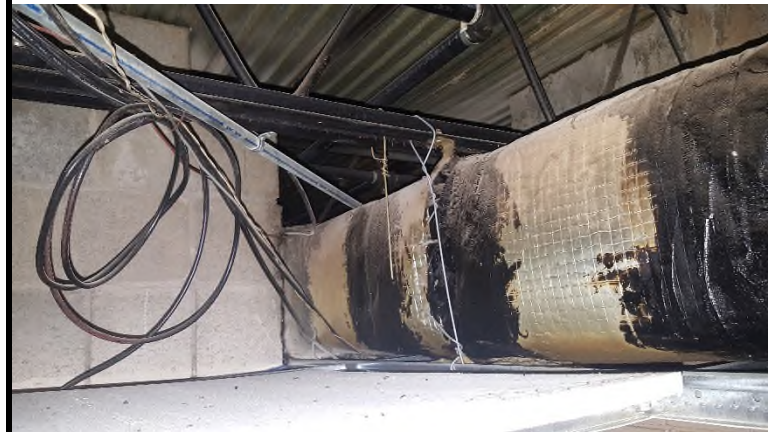
4 The black sealant on the HVAC ducts above the ceiling in the Detention Center tested positive for asbestos (6% chrysotile). Photo taken in the hall near the visitation room.
