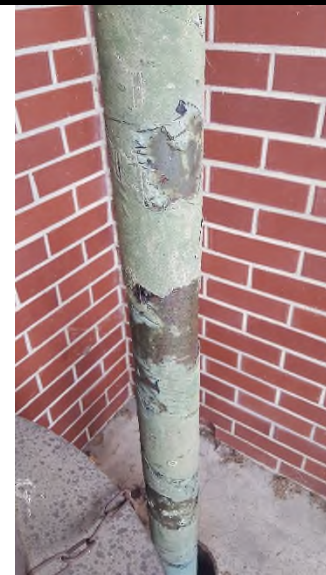
10 The green wrap on the vertical natural gas line on the east side of the building tested positive for asbestos (15% chrysotile).
