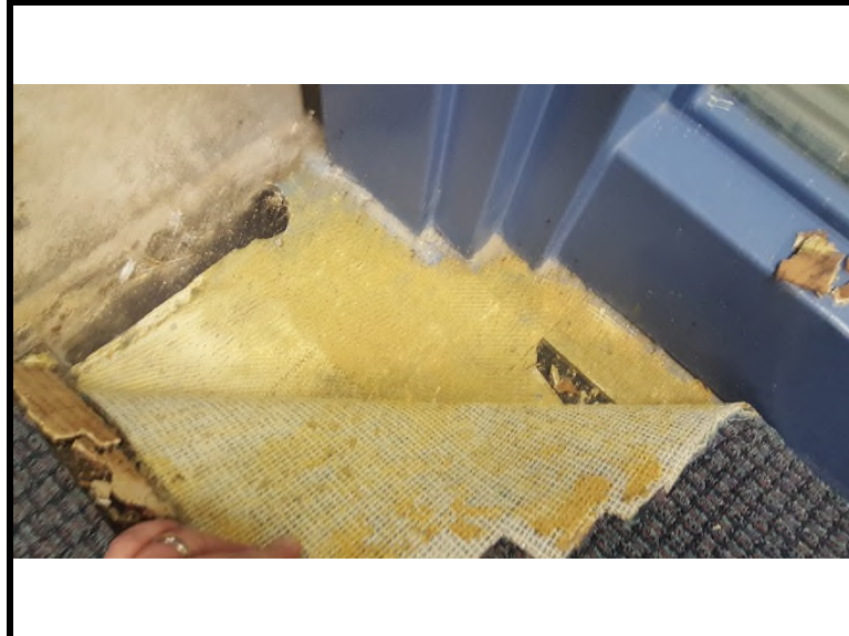
6 The asbestos-containing floor tiles and mastic are present in the Magistrate's side, under the carpet.
