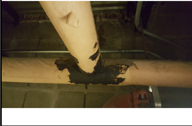
7 The black sealant on the fiberglass pipe insulation above the ceiling in the Detention Center tested positive for asbestos (5% chrysotile). Photo taken in the public lobby.
