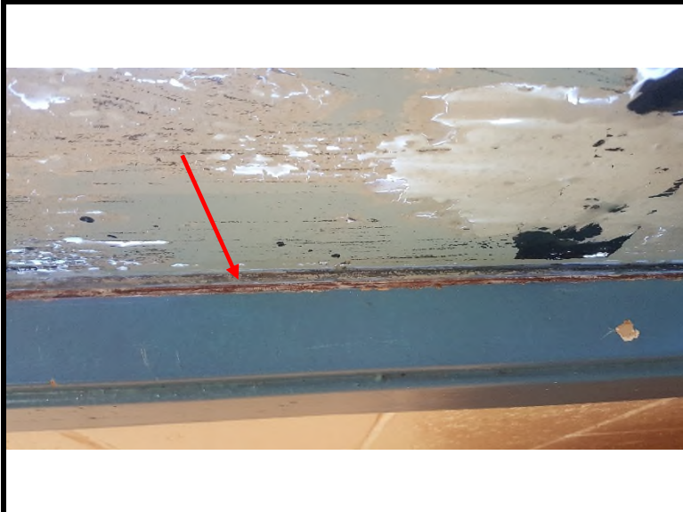
9 The gray caulking located on the inside of the windows between the panes and the metal frame was reported to contain 5% chrysotile.
