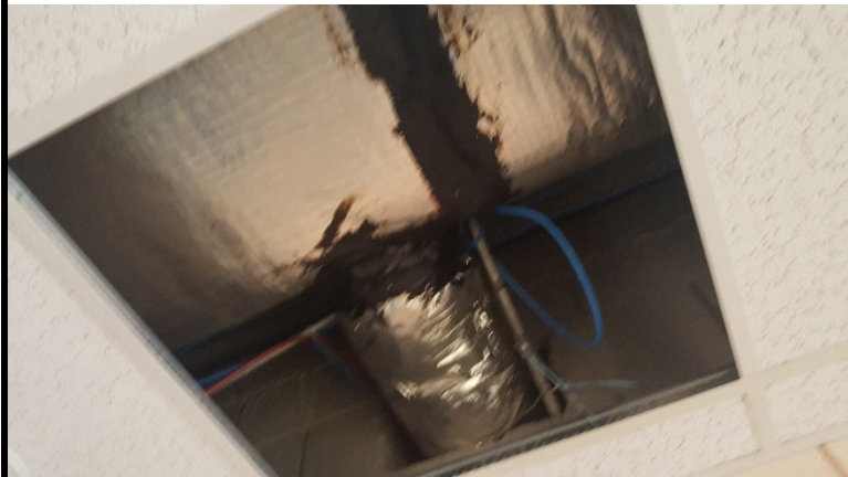
3 The black sealant on the HVAC ducts above the ceiling in the Detention Center tested positive for asbestos (6% chrysotile). Photo taken in the public lobby.
